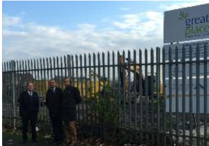
Paul, Ronnie and Stephen at the Old Cricket Ground site as the building work begins
